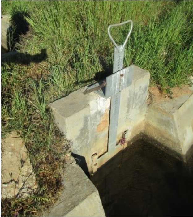
Figure 3.10 | Typical canal off-take
