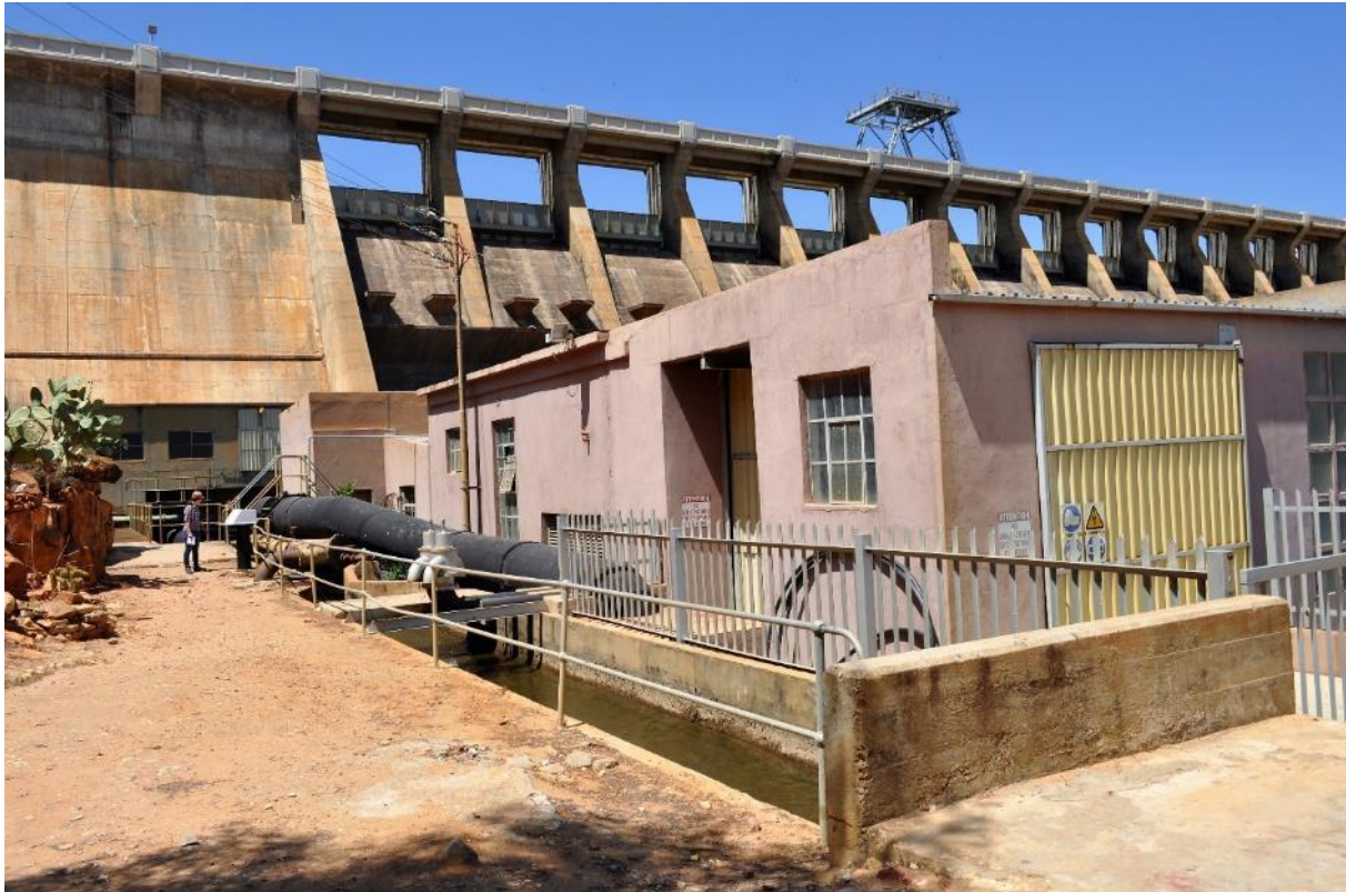
Figure 3.3 | Existing turbine on the right bank of Clanwilliam Dam
